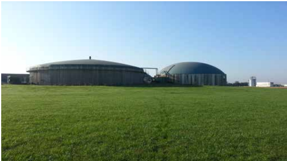
Abb. 1: Biogasanlage in Alerheim (Rainer Weng)
